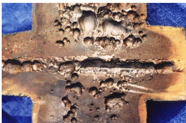
Figure 3. MIC corrosion at girth weld. With suitable data analysis, costly pipeline digs can be reduced by 30 - 50%.
